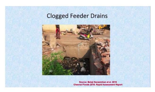
I will show you some pictures. This is a feeder drain which is clogged with solid waste. Definitely this kind of a drain, this kind of canal or a channel will not be able to drain the area very easily and will lead to waterlogging.
