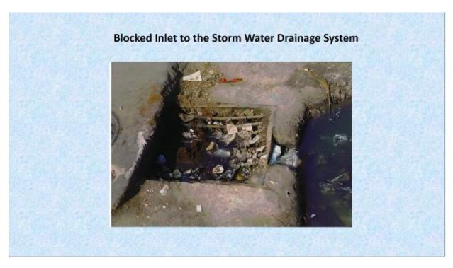
This is another one, here you see this is an entry point to the drainage system, and this entry point to the drainage system again is clogged due to a lot of solid waste. So, how do we expect during the heavy, intense rainfall events, the rainwater will actually go through this into the
