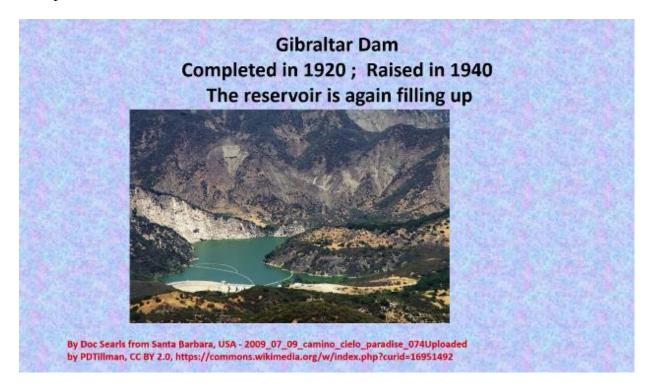
It was completed in 1920. Completed and commissioned in 1920. However, within 20 years that is from 1920 to 1940 within this 20 years because of a significant amount of sedimentation
