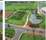
So, it is, these systems you can actually developed as close to a natural echo system as possible, it is. This is one of the bigger one way of very big bigger stuff DEWATS system that CDD has done. This is for Aravind Eye Hospital in Pondichery, which treats about 3 lakh liters of water every day, it is now working for the last almost 10 years of a more I think almost 20 years or something.
