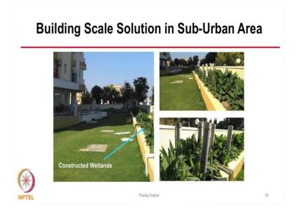
And if there is a space we can have a simple natural treatment system also, which is called constructed wetlands in a scientific language where you have the septic tank at the bottom of the building, again this is a high rise building and this is the basically a septic tank and it can be baffled, multi baffled septic tank also.
