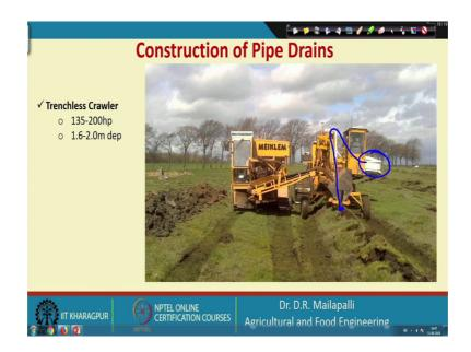
So, the next is trenchless crawler. So, this is also very popular because, in trenchless crawler it does not make any trench ok. So, and it has 135 to 200 hp and 1.6 to 2 meter deep ok, this is the deep And then here if you see, so, this is the cutting tool ok. So, this is the cutting tool. You do not see any trench here, this is all underground ok. So, there is no trench is seen.
