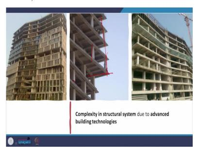
Now, the structural system is complex. That is what I talked about creative and architectural freedom. As you can see, this part of the structural system is very interesting. It is cantilevered out and then the columns are standing on top of that cantilever, and then these floors are going up. So this would have required quite a lot of quite a bit of ingenuity to come up with the form a structural system like that.
