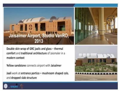
And then we have the Jaisalmer Airport by Studio VanRO in 2013. It has a double skin wrap of GRC jaalis, glass reinforced concrete jaalis and glass itself to provide thermal comfort and also reflective of the traditional architecture of Jaisalmer in a modern context.
