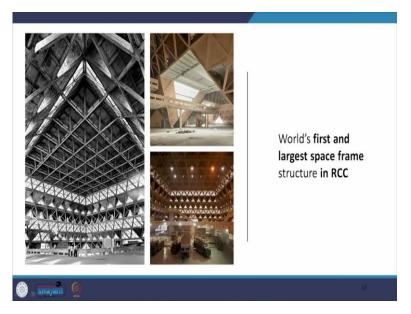
Now, this happened to be the world's first and largest space frame in RCC. Space frame are already being built in the west geodesic dome, many other examples are there.
