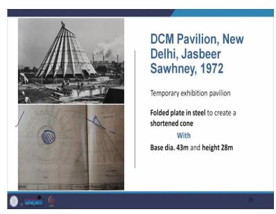
Then again we have folded plates, not in RCC, but in steel. So this was in the DCM pavilion in New Delhi, which was designed by Jasbeer Sawhney in 1972. It is a temporary exhibition pavilion having folded plates in steel to create a shortened cone, that means the cone has been sectioned off from the top. And the base dia of this cone of folded plates is 43 meter and a height of 28 meter.
