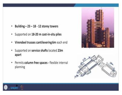
So we have the 12 meter high, 18 meter high, and the tallest is the 23 meter height tower, and this is supported and cast-in-situ piles. The Vierendeel trusses are cantilevering outward 6 meters from the end, these are the shafts of the building, the shafts have been provided. As you can see these are the vertical shafts of the building service shafts of the building, which
