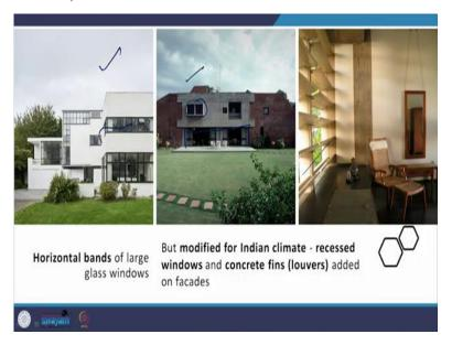
Then the horizontal bands of large glass windows as you see here again made possible because the outer wall is only a curtain wall, so it is not carrying any load. Now, the same thing does not happen here in this house simply because it is in India and for it has to be
