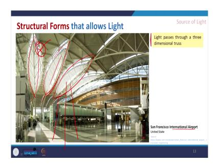
This is another wonderful example from San Francisco international airport where the whole structure is being made with the truss frame and in this you can get a very nice combination. So, this kind of folded, this boat like structure is also giving a sense of a petal and this is giving a nice view of the roof as well as essential functionally it is giving some light inside.
