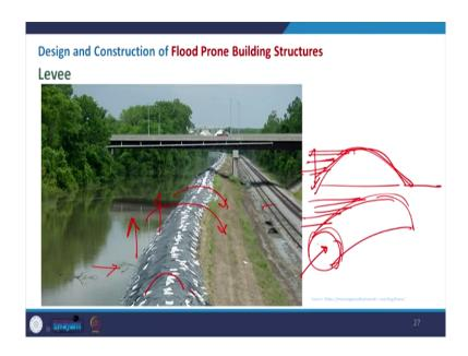
So, here you can see that this is a railway track and there is some water body and this is being protective. So, if there is increase in water during the flood. So, this will initially help to not you know overflow this water to this site. So, this is the profile is being maintained like this.
