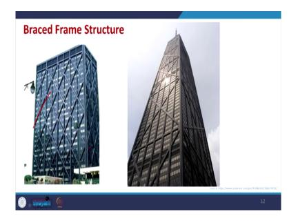
So, coming to the braced frame structure: so, in this case along with the frame we have some structural bracing. So, you can see that this building or this building you have some vertical structure along with that those are connected with some additional bracing which will help this building to protect against the lateral load.
