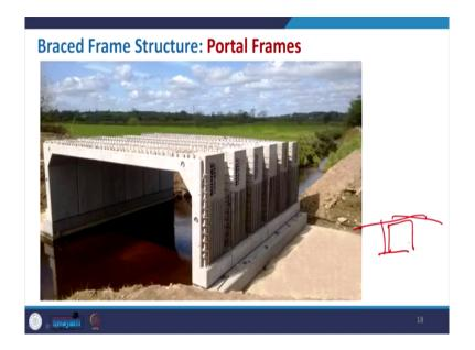
So, in this case this is not made of steel, this is just with the concrete the shear wall kind of construction. So, this is just creating to you know underpass to pass this particular water or the candle they have. So, this kind of arrangement, this kind of bridge sometimes we need the portal and if you compare it with this steel representative portal to this, it is pretty similar and that will actually helping to make it.
