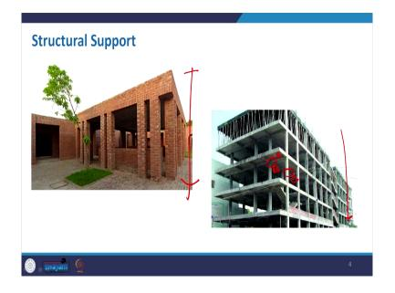
Now, in this case, I have you know given two different pictures side by side and I just want you to guess like what could be the reason to put this, ok. So, maybe you can find it out very easily where it is something a very low; low height structure and made of brick masonry, you cannot see any such concrete column or something like that fully made of brick.
