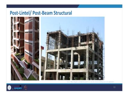
So, here you can see two examples where this is very clear that we cannot see any wall on it and still it is stable and still under construction and this is the finished building. So, this particular wall is just giving some protection, some privacy for the interior space and this you know particular opening created at the top is giving light or ventilation inside, but basically overall it is the post lintel structure.
