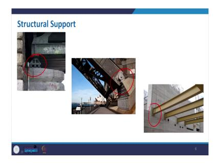
Now, in this case in order to make it more clear to you, this is the example of a breach at the one support you can see, this is a roller type support. A joint in one end where this is the other one this is your pin joint and here it is fixed to the wall and neither of the pin or roller it is basically the rigid joint. So, depending on that also we will have the arrangement.
