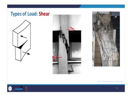
So, that we put pressure in the different direction and then it got the results. So, here two pictures that you can see this is again a failure of column due to shear. So, it is moving this direction and this direction and it also depends on the rigidity or stiffness of the property will come into the later stage to discuss it.
