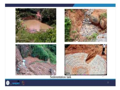
We need huge areas where the water can be, the entire water from the site during a storm can be brought; it will be allowed to stay there, retain. It helps in charging recharging the groundwater, because the water will percolate down and it will control the soil erosion.
