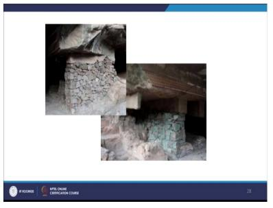
And similarly, they also given some support systems where there has been cracks and there is a possibility that this may not bear the load after some time that is where they started giving some kind of huge rubble masonry wall, not masonry, it is a kind of dry stone wall which they have able to give a little support on that. So, without giving any additional material or a render to it but just keeping as a stone wall.
