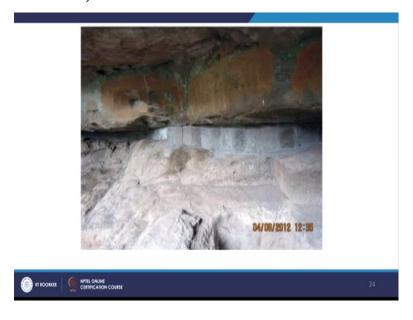
So, now you can see that they have started looking at how the edges of the roof and the structure of the vertical aspect and the roof aspect are merging that is a lot of damage have occurred, and there might be a chance that it might collapse at any time. So, that is where they started giving some kind of support system at the edges so that there is a you know the balance of the structure as well.
