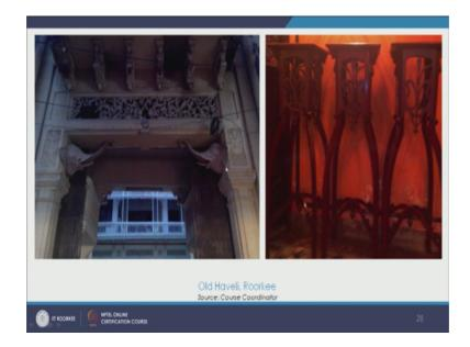
We see over here this elephant and this works as a bracket over here, here it works as a bracket. We see some stone work here which has been broken now we see these brackets.
