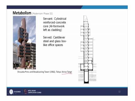
Which is again designed by Kenzo Tange in Tokyo the capital of Japan, here also you can easily understand, this is the service servant spaces, which is a cylindrical reinforced concrete core. And the core is reinforced concrete, but what we are seeing is the form work, we will discuss the form work that the concrete form work which they used to take
