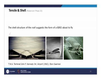
Now, coming into the examples of the tensile and shell structure; So, this is a shell-structure design by Eero Saarinen which is around 19 which is in 1962 this is in New York. So, as we are discussing the shell structure gives the form which suggests that there is a BIRD which is about to fly or just landed and if you look at the building.
