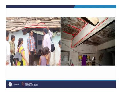
Here, you see there even the roofing material is a very thin slabs if you look at the girder the stone girder, here and then these stone slabs have been and then they filled with a kind of lime mortar or something like that.
