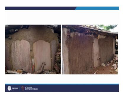
And you can see the finishes, how they are joining with this cow dung and the kind of slurry. What they get? And the finishes it is almost like a kind of wattle and daub construction.
