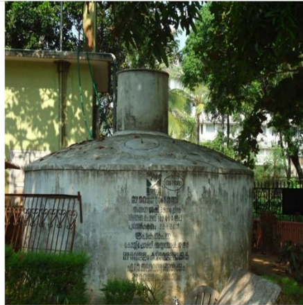
A 35,000 litre rainwater harvesting tank in Kerala Source: Wikipedia
