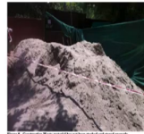
Figure 8: Construction site showing soil and material management
