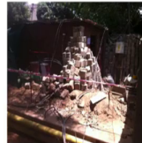
Figure 7: Construction material has been recycled and used for project
