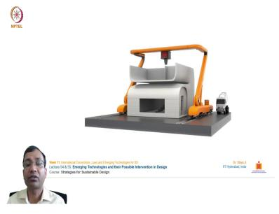
This you must be aware of like a 3D printing it is a like additive manufacturing actually technology. So how this 3D printing is also adding to the like a construction of like a like an efficient way plus it minimizes a huge amount of like a waste you know because it does not leave any like a residue or any like a extra actually material it lays only material where it is necessary or whether where it is designed to be laid.
