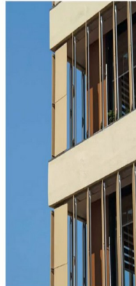
Louvers can be used as a building element to cut down on the sun while expressing them as part of the external facade
