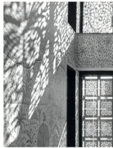
Jaali as a form of fenestration allowing for breeze and yet cutting on intense sun while offering play of natural light
