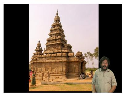
In fact the first free standing temple, so this is now a constructed temple at Mahabalipuram not carved out of a single boulder but made up of different stones. The short temple as it is called is made up of these long shalas and these square kutas at the ends. Note, there is no amalaka on the top but a big hut.
