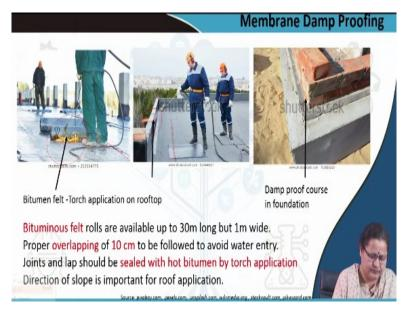
So let us see how the conventional material that is bitumen sheet is being applied. You can see the picture where a person is actually rolling out and there is a fire burning underneath. So this fire is helped to melt the bitumen so that the bitumen sheet gets stick to the surface onto which it is put.
