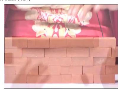
So, this is a 5-inch thick wall. This is the first layer, and I want this end to be flat. So, as per principle, we have to start with a full brick such that this joint (line) does not appear. If I would have started like this (see video), then this part would have
