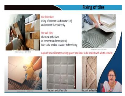
After knowing all these, you also need to understand how to place the tile in position. The given pictures are illustrative. A serrated (grooved) base is made. Similar serrations are made on the walls too. This pattern is made using a specialized trowel. Thus, something is spread on the wall, on top of which this tile is fitted. These photographs are taken from the back of the tiles.
