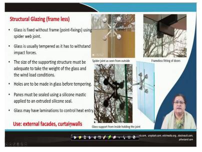
We will now discuss the structural glazing or the frameless glazing system. In the pictures here, you can see the 'spider joints'. These help to fix glass at intermediate points, without the need for a frame. The views of the assembly (after installation) from the front, back, and sides are given (see images in slide).
