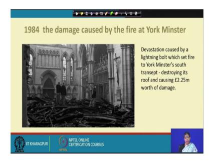
The devastation as you can see the devastation caused by a lightning bolt it happened due to lightning. So, nobody can help that, which set the fire to York minister's south transept and it destroying, it is roof the entire roof collapse and causing the 2.25 million of pounds worth of damage and, this is the scenario which happened.
