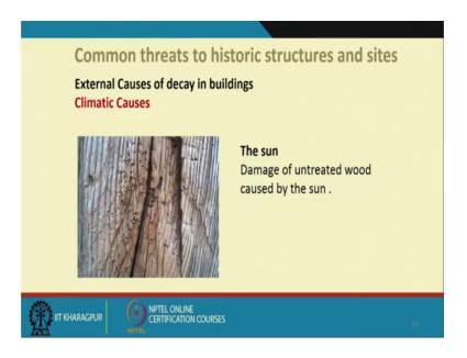
Due to the sunlight the damage has been taken place in the untreated wood, which is caused by the sun because the wood is not in the very good stated, it was untreated. So, the sun light can also cause the problem. Now these are the various sort of a manifestation which the climatic reason can happen.
