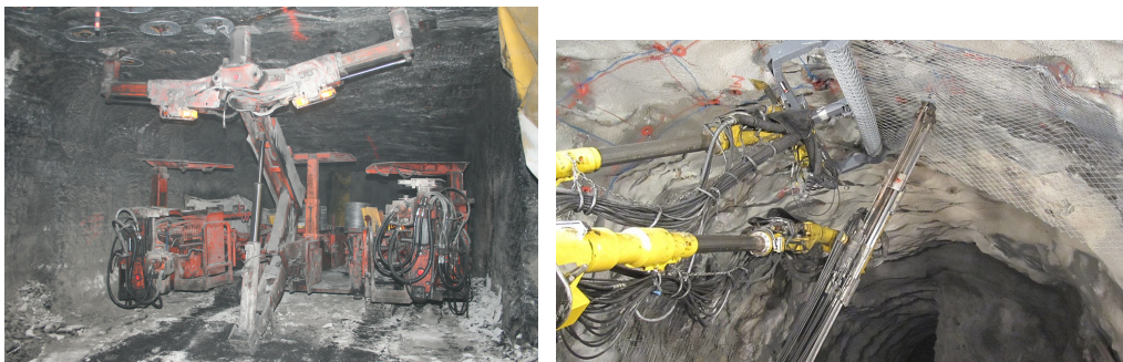
Figure 4. Scaling and supporting equipment's
