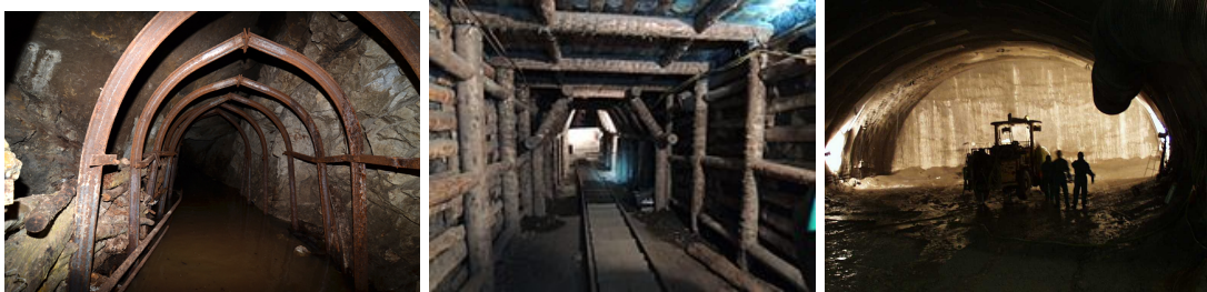
Figure: From left- “D”, “Rectangular”, “elliptical” shape of adit
