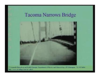
What you saw over there was a bridge; the Tacoma narrows bridge collapsing. The bridge collapsed because of resonance. There were very strong winds in the place where, the bridge was located and these winds had a time dependent oscillating part to it. So, those winds were not the wind was a not a constant wind, but it fluctuated with time. And this fluctuation in time had an oscillating component, which matched with the resonant frequency of the bridge.
