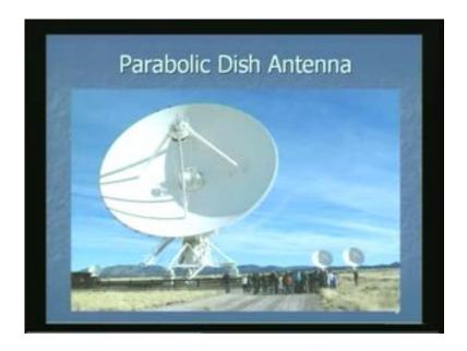
The Electromagnetic Waves get focused on to this point and then it gets converted into electrical signal and that electrical signal is processed further. The same dish will generate electromagnetic wave if the electrical system is supplied to the feed, which will get reflected from this and it will get into the Space.
