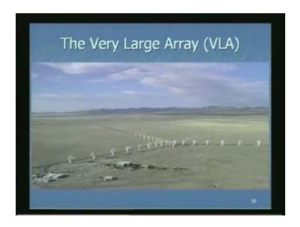
This dish is of the diameter 25 meters but the total spread of the antenna is of the order of 21 kilometer and therefore we get an effective aperture which has a radius of 21 kilometer though each antenna has a diameter of only 25 meters.
