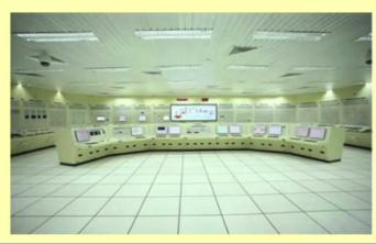
Simulated Sub Systems include Neutronics, Primary and Secondary Sodium, Safety Grade Decay Heat Removal, Core Temperature Monitoring, Steam Water, Electrical and Fuel Handling System.
