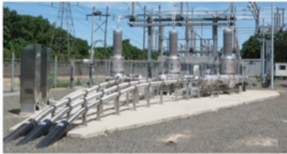
The world's first high temperature superconductor power transmission cable system in a commercial power grid was energized on April 22, 2008 at the Holbrook substation on Long Island, New York, USA. The 138,000 volt (138 kV), 7,000-foot (~400 meter) cable system, the longest superconducting cable in the world, includes three phases connected to the Long Island Power Authority's (LIPA) grid through six outdoor terminations.
