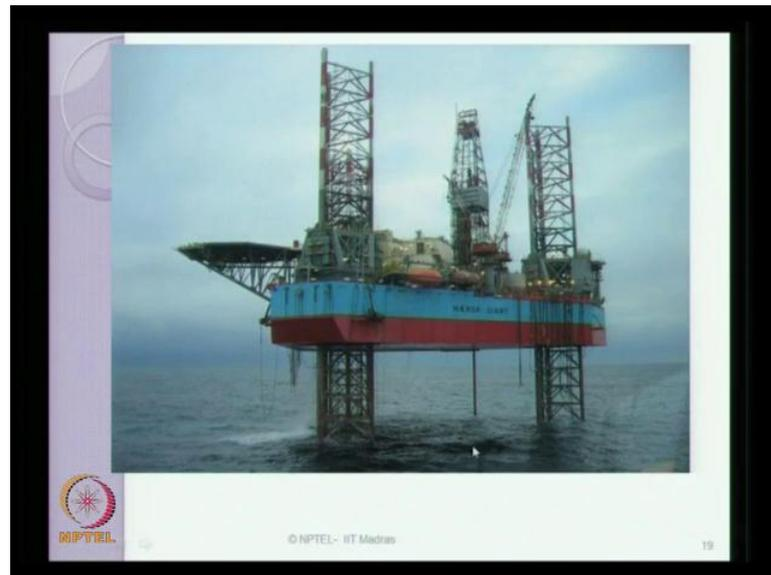
This is a closure view of one of the jack up rig, which is very famously deployed in North Sea, which is Marx Jain. This will give you a very clear picture about, how these legs are protruding the deck and how they are projecting into the sea floor as you see here.
