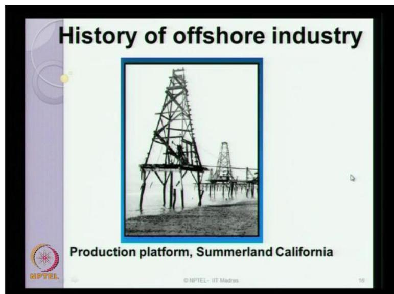
Successively, different elemental production platform are constructed essentially can see that truss type structure, which has been constructed in the early stages. The structures look very simple, resting on four or six columns, which are simply diagonally braced and they were the structures required in initial stage, when the water depth of exploration was very shallow. We can see there are series of structures, so offshore industry on the
