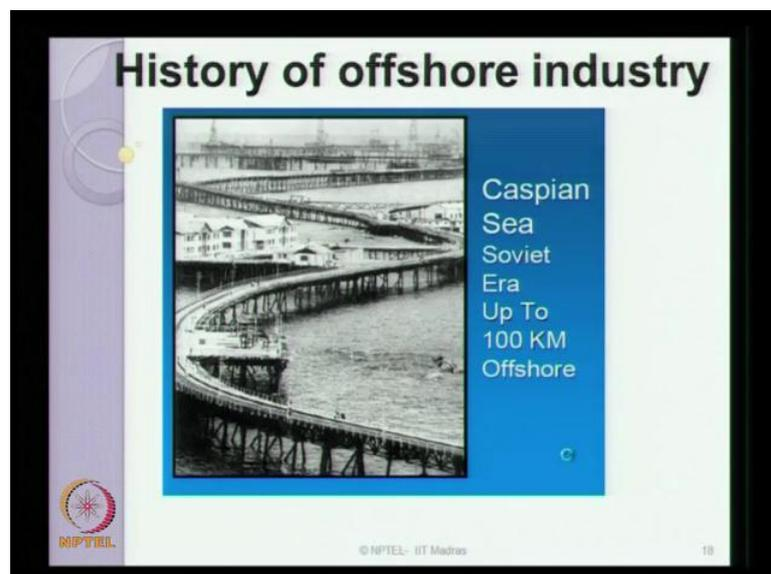
Similarly, in Caspian Sea Soviet Era up to 100 kilometer offshore, we can see there are lots of derricks constructed and an approach load has been made to transport the oil explored in these sides to an onshore area.
