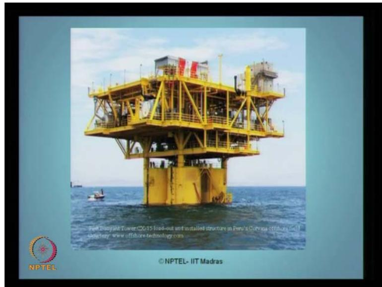
Subsequently, a platform was attempted as a tension buoyant platform, the first buoyant tower CX 15 was loaded out in the Feru carnivo offshore field, which has now become a promising figure, which is going to now produce oil end of 2013. It is the new platform, which has been constructed recently, which is commissioned now.
