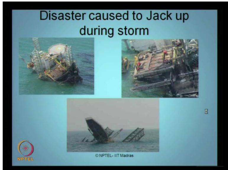
As I said, disasters can be caused to jack up rigs during storm. Here is a photograph, where the complete jack up rig got capsized because of the storm weather. You can see, a complicated top side; we can see here, the three lattice legs; you can also see here, the three lattice legs completely over topped and fully capsized. So, strong and severe storm weather can cause disasters to the jack up rigs; you may lose the whole facility under such kind of critical situations.
