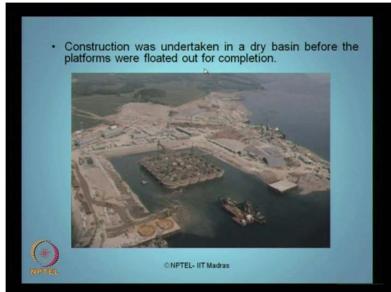
This is the closer view of the platform. You can see here, the caissons have been constructed and then they have been tucked off by the board. The construction was undertaken in a dry basin, as you see here, before the platforms are floated out for completion.
