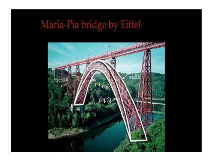
There is also when you have the topology next thing is the shape here you see, the shape of a bridge that was designed and built by Eiffel had a depth which was varying from end to end and so, was the width in a different way that the shape optimization and of course, the cross bars and cross bar, even cross bar is also evident here of this hierarchy that we can talk about.
