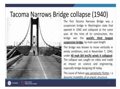
So, these are the flutter we can easily see under the influence of the air or the wind, it was fluttering up and down and this under the extreme conditions led to the collapse of the bridge.
