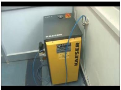
So this is a tube pipe from which compressed air is coming from the compressor, so this is the Kaeser compressor, it is refrigeration type air compressor, it is 100 percent moisture-free that is a not going to harm the machine. So the compressor that we have to use here, it has to be moisture-free.
