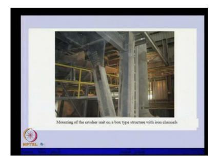
So, if we see from bottom. So, this was the support to mount that machinery at the top. They had lot of vibration in this of order of vibration was very large because of that even in the columns. So, whatever this kind of columns, they had the cracks in the columns. The machine was in very bad condition. They did not know what the actual cause of such vibration was.
