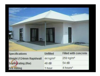
Now in this slide, you can see a house built with the help of GFRC panel, and builds specification of the house is shown. Now, moving on to the process of erecting this
