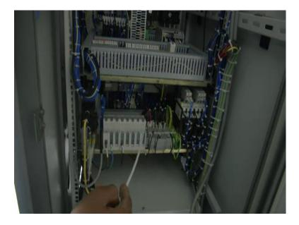
Then, see it is for sometimes if some selective switches will not be getting numb on that time, we have we have to troubleshoot. On that time we have to observe MCBs also. Suppose some MCBs are the tripped or what like the type. And this is called a contactor and thyristor 24 DC is supplied, this is for control circuit um. We given two numbers of control tray: one and two numbers um. Then there are also power supply.
