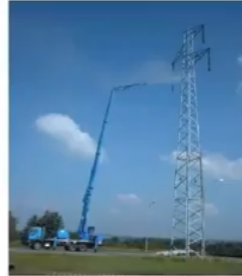
Fig 9 : Telescope Boom Insulator Washer
