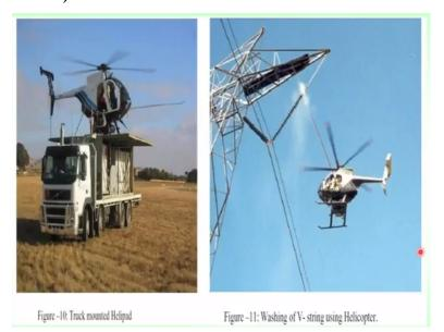
This are again the tuck mounted helipad where it is being used for the cleaning of insulators. **(Refer Slide Time: 26:33)**
