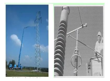
This causes lot of revenue loss for the utilities this is one of the again example of the telescope boom insulator to cleaning method used by few utilities his is live line washing method. (Refer Slide Time: 26:21)
