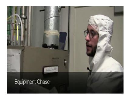
The first you think to check in the gas rooml the gas chase is like the CDO box the CDO box is responsible of neutralizing the exhaust gases from the STS.
