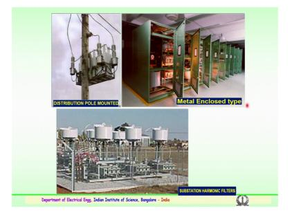
Similar examples are connected with the capacitor banks. So, several types again before the distributed pole mounted you have arrangement of the distribution system. This is metal enclosed type of a capacitor banks which are arranged in a typical substation, along with the capacitor bank you have the harmonic filters and in a EHV or a UHV substation. So, these are various types which are capacitor banks which are being used for the proper correction of the power factor.
